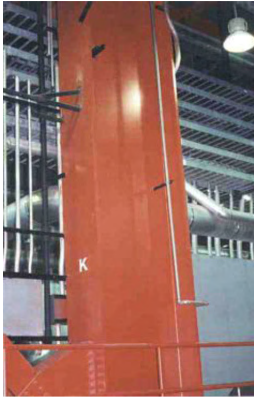
Figure F-2. Typical support column in the Turbine Building.
